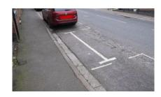
H bar road markings are to deter parking over driveways and other vehicle access points. Obstruction can result in a fine
